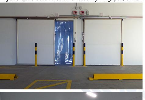
The door package consisted of: 2 large sliding doors to allow for forklift access, a chilled hinged door for access between the rooms and a 1 hour Robust fire door, leading out to the fire corridor.
